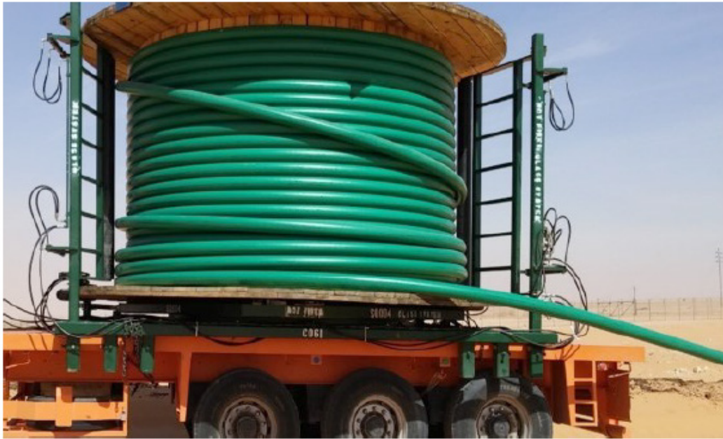
Figure 2. Installation of spoolable reinforced thermoplastic pipe. (Courtesy of Saudi Aramco)
